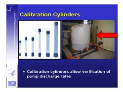
Calibration cylinders installed in the piping manifold allow pump discharges to be checked so that flows are accurate. This is particularly important with fluoride, as the flow rates tend to be very small.
