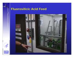
It is recommended that the storage tanks be enclosed in a designated room. This installation has a view window so that key controls and operations can be monitored without entering the room. This room also includes a depressed floor to provide firm spill containment in the event of a leak or spill. Not all treatment facilities have such a containment, but if your facility is considering an expansion or redesign, this is something to consider.
