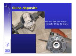
Here are examples of silica deposits within pipes if the wrong dilution occurs. In one case, the strainer is clogged. In the other, the pipe scales. Remember, most waters have from 5 to 30 mg/L of silica, so there is a another source of silica that just from the FSA.
