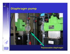
Diaphragm pumps have an oscillating membrane head, which alternately sucks the solution into the pump and then discharges the solution. Inlet and discharge check valves ensure that the fluid moves in one direction. The diaphragm pumps have a replaceable head, which should be replaced annually as a preventive maintenance measure. Also, the check valves need to be inspected and replaced if necessary.
