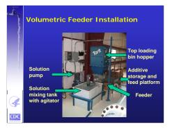
Here is another feeder installation. It has a slightly larger bin hopper, and there is a loading platform so the operator can have easy access to the bid feed location. For even larger facilities, the bin loading location might be on the floor above the one with the hopper, or you can get bin loaders with elevator lifts as part of the bid loading so the bags can be added at ground level of the building.
